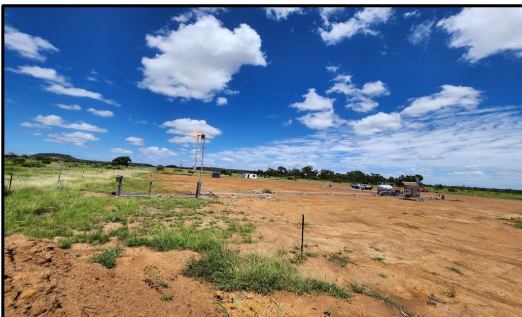
Figure 2: Gas flare during commissioning of Sapphire 5 L lateral wells: Source: Blue Energy
